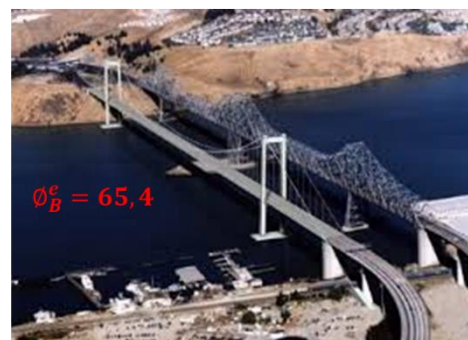
Carquinez Strait bridge, California USA (1927)
